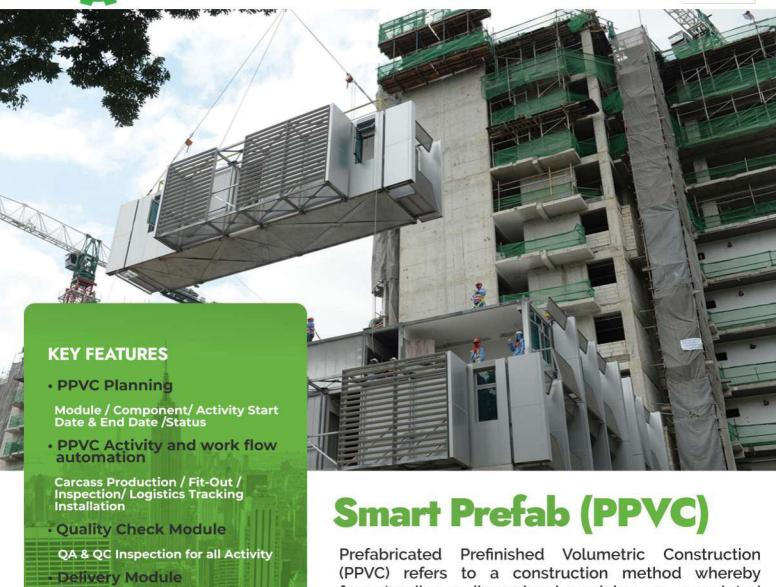
Prefabricated Prefinished Volumetric Construction (PPVC) refers to a construction method whereby free-standing 3-dimensional modules are completed with internal finishes, fixtures and fittings in an off-site fabrication facility before it is delivered and installed on site.
